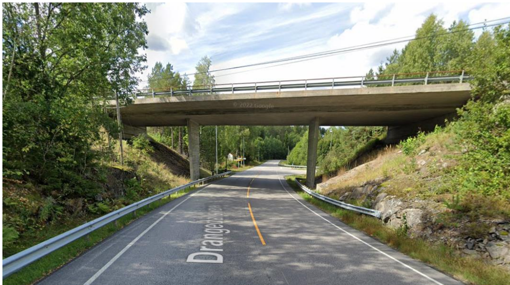
Figur 3-14: 08-0919 Gjerdemyra bru. (Foto: Google Street view).
