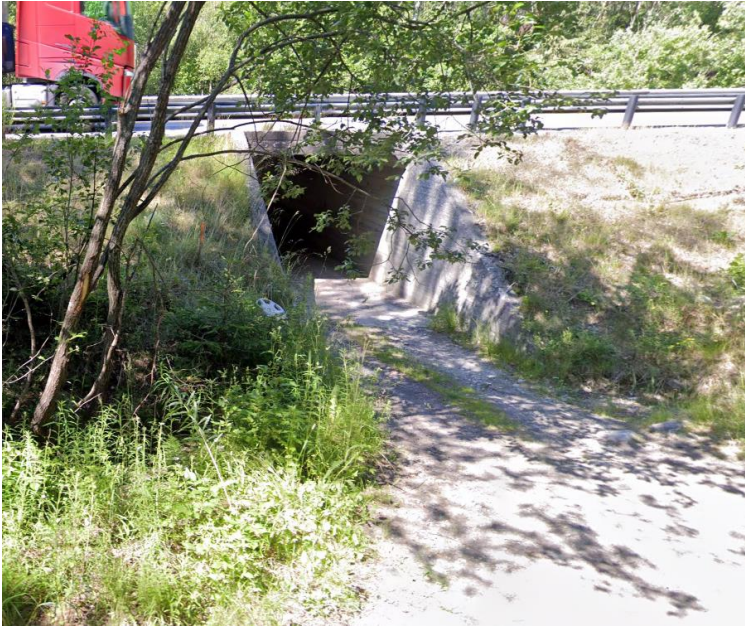
Figur 3-8: Eks kulvert. (Foto: Google street view).
