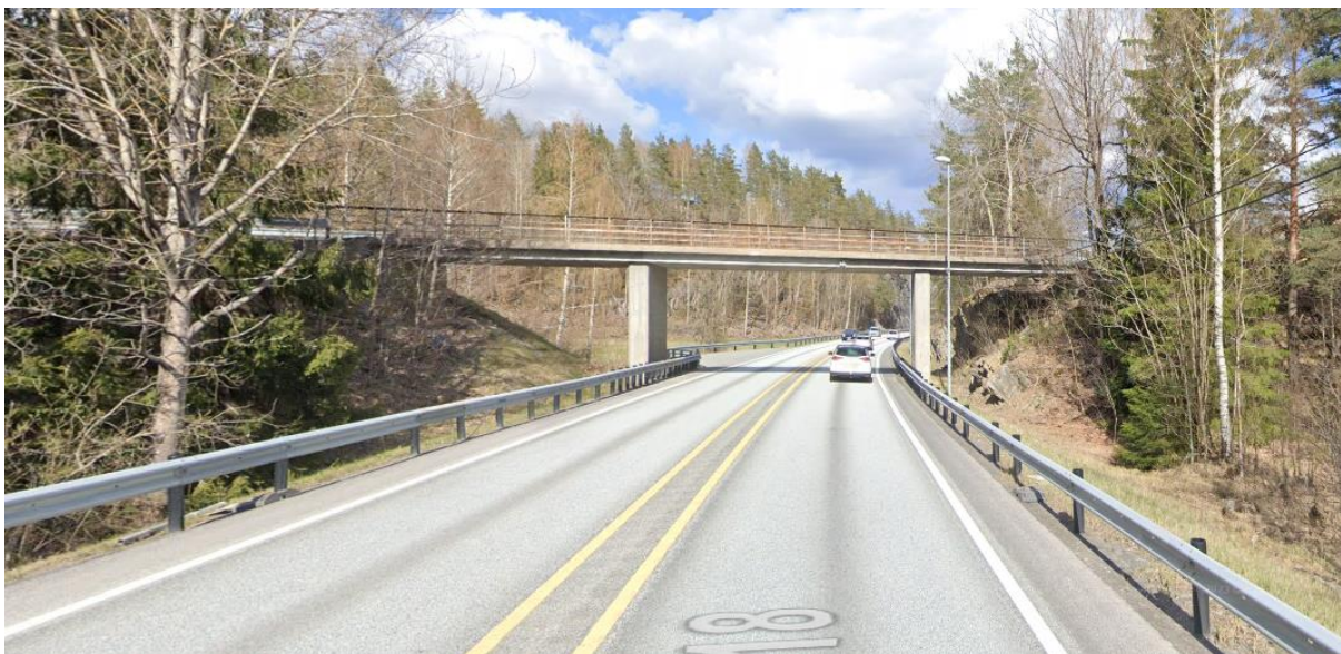
Figur 3-34: 08-0763 Setern bru. (Foto: Google Street view).
